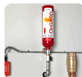
Fire Suppression (Water, Halon, CO 2 , LN 2 )
